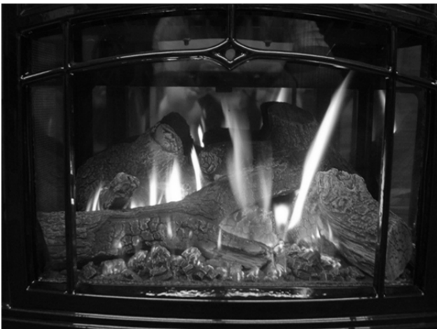
Photo 9 – Typical Burner Flame Appearance
