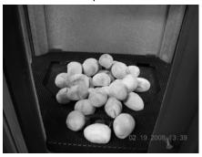
Install 10 stones on the second layer, filling in spaces in the lower level. Distribute the stones evenly over the burner. NEVER stack the stones more than 2 high
