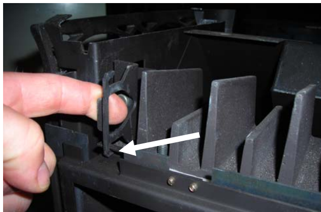
Photo 12 – Glass Spring Clip Detail
