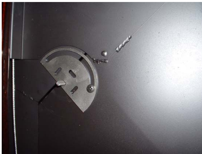
Photo 13: Restrictor Fully Closed
