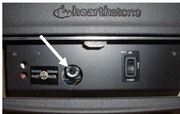
Photo 39 – ST Valve Output Control
