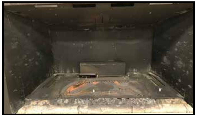
Figure 3 Base Refractory Installed
