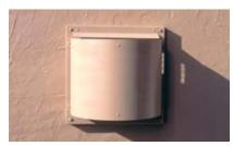
You can enjoy the convenience of a gas fireplace anywhere in your home with a **Regency Direct Vent Fireplace**. Regency Direct Vent Fireplaces maintain indoor air quality by drawing fresh combustion air from outside through our specialized venting system into a sealed firebox and sending the used air back outdoors.
