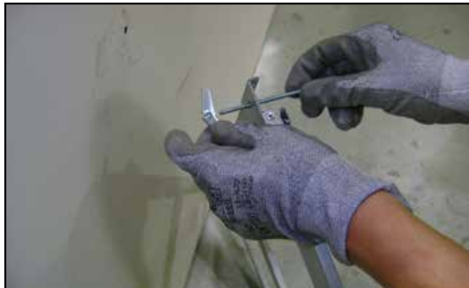
Figure 4.10 Toggle Bolt Installation through Mounting Bracket
