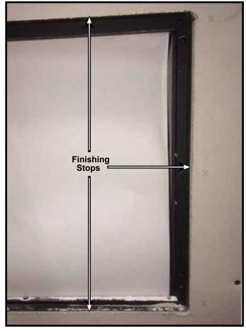
Figure 4.5 Wall Finishing Stop Locations and Dimensions
