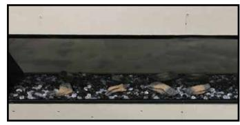
Figure 4.10 Media and Small Logs Installation
