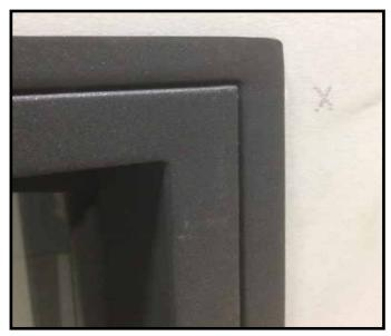
Figure 4.7 Front / Trim Ring Installed to Overlap Wall
